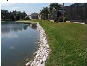
ponds within the community. The objective of the project was to restore the eroded banks to the permitted side slopes and repair drainage structures required for safety and functionality. *(Construction performed to-date: \$450,000)*
